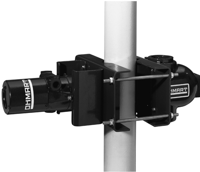
FIG. 6.6g Actual installation of a densitometer.
