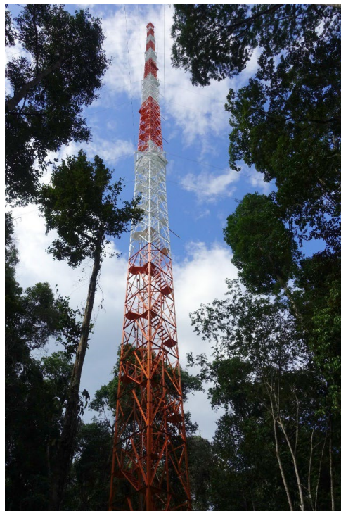
Figure 5.1.1 – The ATTO 325 meters tall tower in Central Amazonia. Aerosols and trace gases are being measured continuously at the top of the tower and profiles for trace gases and particles.
